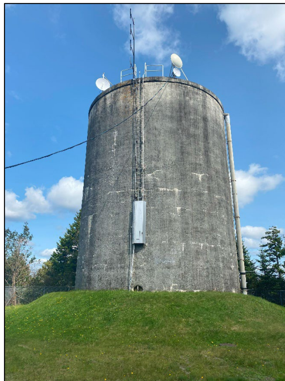
French Village Water Tower
