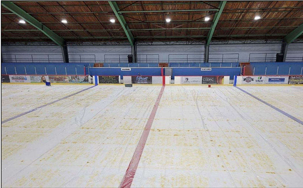
The middle ice surface, covered in the with plastic to protect from condensation dripping from the ceiling.
