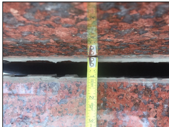
Photos from a Survey on the Monument showing the disconnections of base and seems
