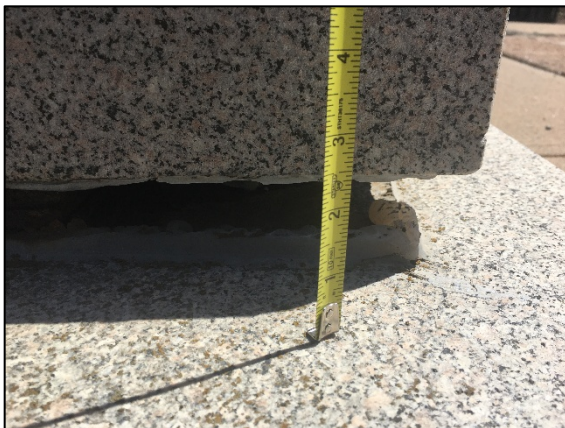
Photos from a Survey on the Monument showing the disconnections of base and seems
